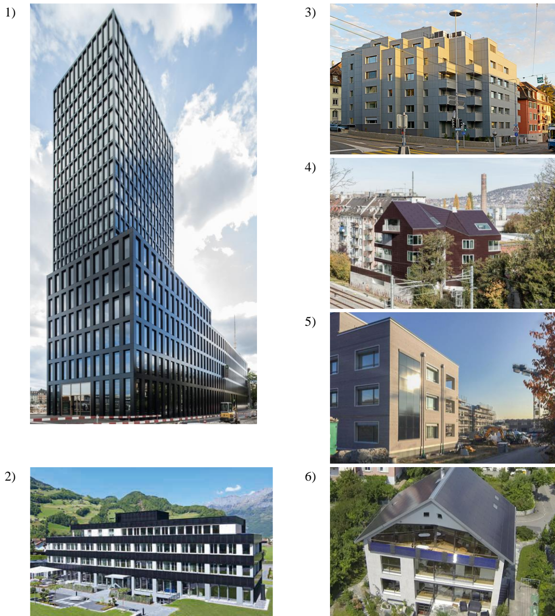
Fig. 3.1 Photographs of the selected buildings with integrated PV systems: 1) Grosspeter Tower, Basel 1 ; 2) Flumroc, Flums (Flumroc 2015); 3) Viridén+Partner, Zurich 2 ; 4) Solaris 416, Zurich 3 ; 5) Setz, Möriken 4 ; 6) Rudolf, Thun 5 .
